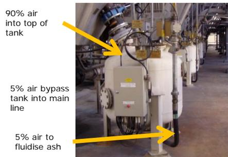
Figure 2: Flyash Blow tank feeder airflow improvement into pneumatic conveyor
