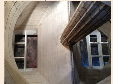
Figure 2: Installation of baffles into the two legs of the transfer
