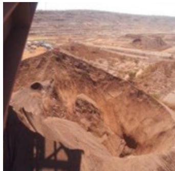
Upgrade of Iron Ore Gravity Reclaim Stockpile to increase Live Capacity. a) Rathole formation reducing live capacity; b) Post-modifications stockpile drawdown
